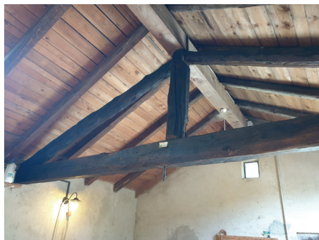
Caset, capriata in restauro
